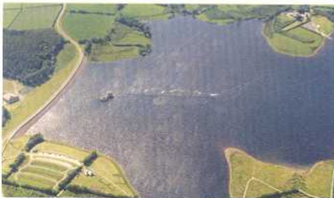
A destratification system is in place at South West Water's Roadford Reservoir.
